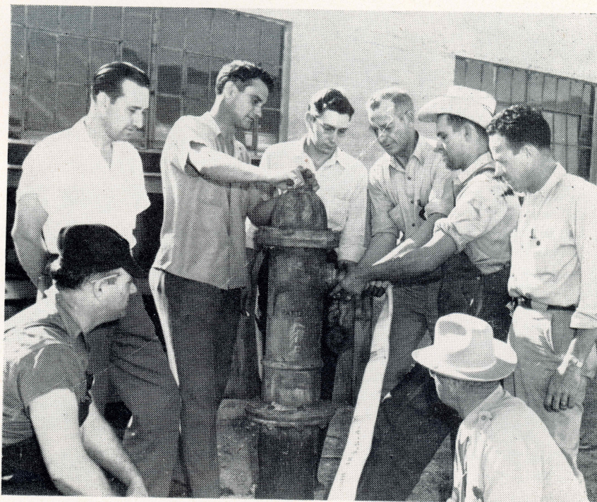
FIRE BRIGADE CREW —Practicing for any emergency that might arise, this volunteer fire crew taps a plug under the direction of J. G. Pearce, left, of Sheet Metal, assistant fire chief, and C. A. Addington, right, of Plant Protection, fire chief. The others, left to right, are J. M. Nichols, Ed Hukill, C. M. Duncan, M. W. (Hap) Herring, R. W. Wills and C. E. Yarnell.
