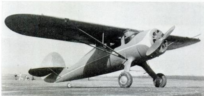
It is quite evident from the general design of the Phantom that Don Luscombe once was a Monocoupe designer and official. The Phantom, however, is bigger and also is all-metal.
